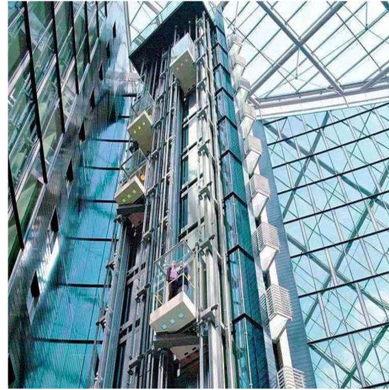
Fig: 2 - Modern elevator
